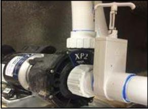
**Slide Valves:** Valves are used to shut off the water flow to the heater, circulation pump, Secondary pump, and Fitness pumps for specific service problems.
