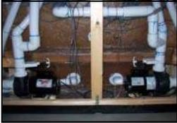
**Fitness pumps:** Fitness pumps are designed to power the Elite Pro™ jets in both the swim and fitness units. Refer to the Control Section of this manual for detail on programming custom and pre-programmed workouts maximizing the aquatic exercise experience.
