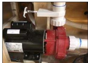
**Circulation Pump:** A dual speed pump designed to use low speed for water filtration and heating and a high speed for hydrotherapy. The jets one button on the topside control will activate the circulation pump. The FX219, FX219s, SX219 and SX219s will have a second circulation pump for the spa zone.
