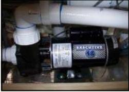
**Secondary pump:** A single speed secondary pump has been added to the hot tub zone of the dual zone models for additional relaxation and therapy.
