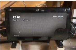
**Support Pack:** The control system operates all functions of the swim spa. Make sure your electrician connects the power supply accordingly to all National Electric Code, and shows you how to test the GFCI circuit breaker (not supplied). This pack is connected to a 50 amp breaker and for dual zone products; FX219, FX219s and TSX 219, there will be two packs, one for the fitness zone and another for the spa zone.
