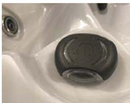
**Air Controls:** Fittings mounted on the lip of swim spa controlling amount of outside air mixed with incoming water of the hydrotherapy jet. Your swim spa has multiple air control on the swim spa lip that control air/ water mix for a segment of the jets. You choose the strength that best suits you. When not in use, the air controls should be kept in the off position.
