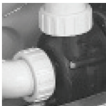
Vent air by slightly opening pump unions.
